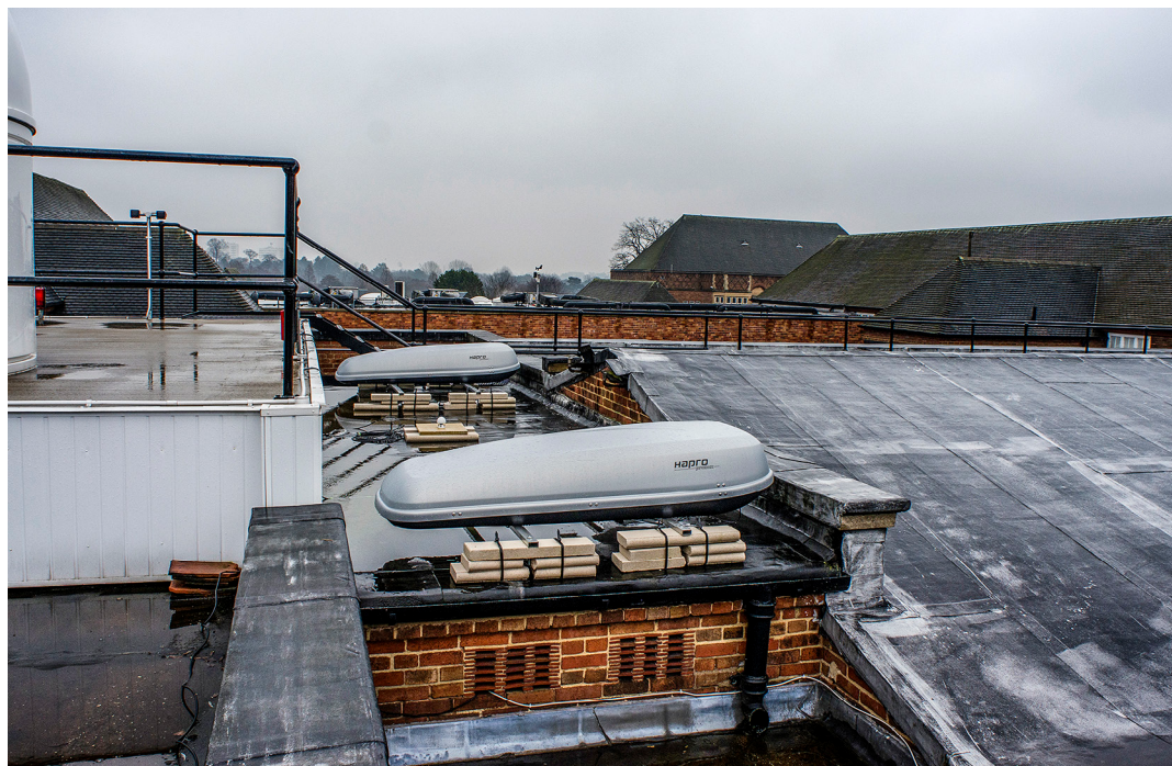
Figure 4 The ski boxes containing the HiSPARC detector, fixed firmly to the school roof
